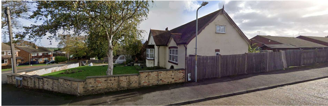
Existing low wall and fencing to be retained, with wall only removed to create entrance to driveway
