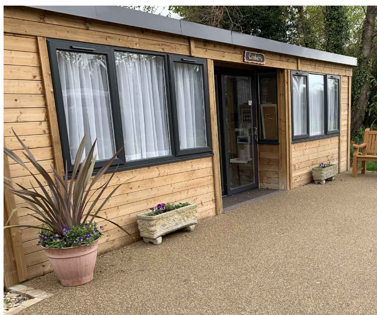
EXISTING GARDEN HOUSE PHOTO 1
