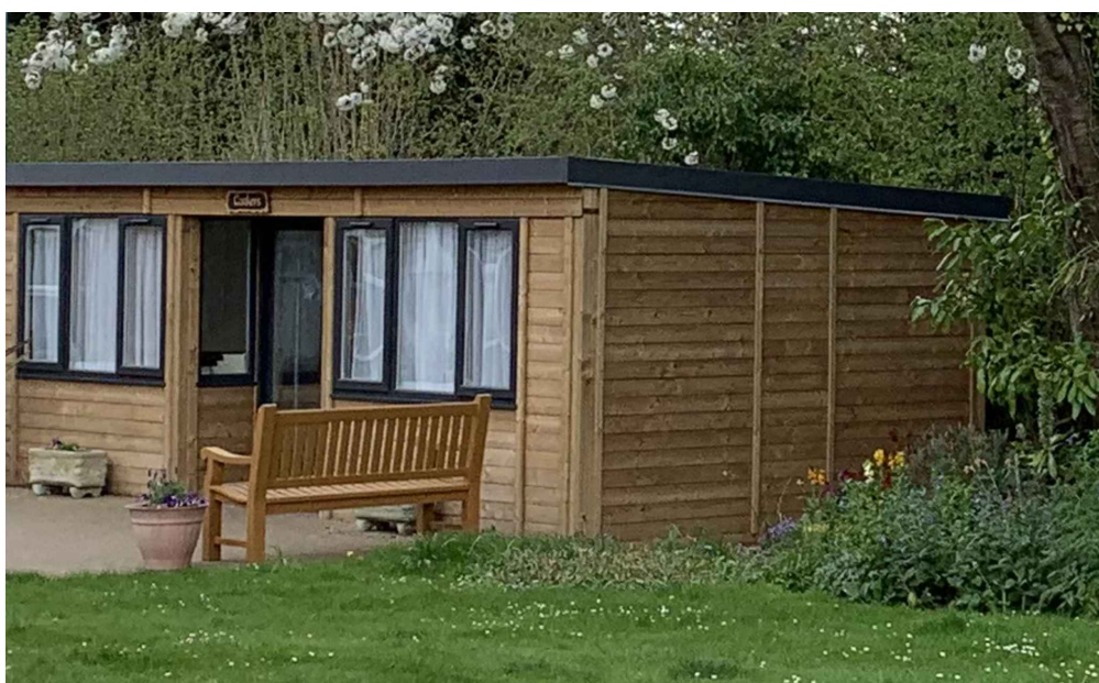
EXISTING GARDEN HOUSE PHOTO 2
