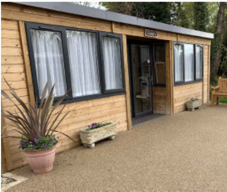
EXISTING GARDEN HOUSE PHOTO 1
