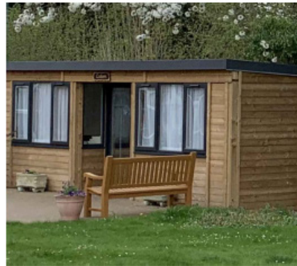
EXISTING GARDEN HOUSE PHOTO 2
