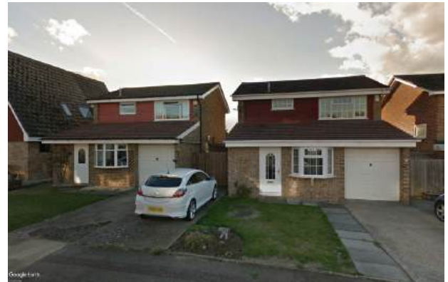
Dwellings containing bay windows and gable end pitched roofs
