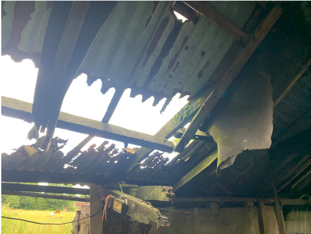
Plate 3 – Section B Truss damage on Gridline 4
