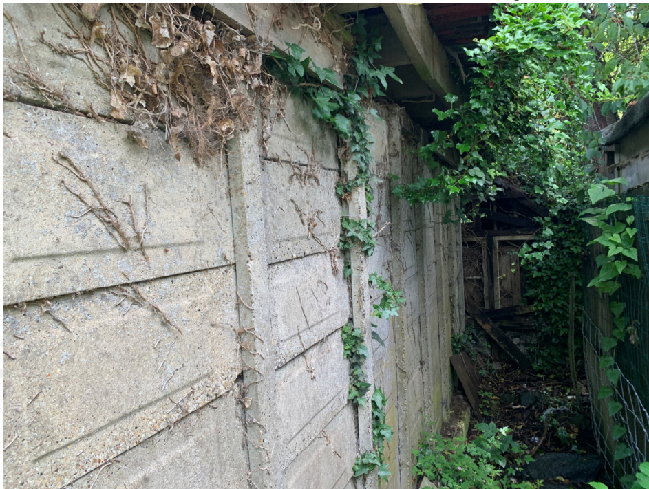
Plate 6 – Section C concrete panels
