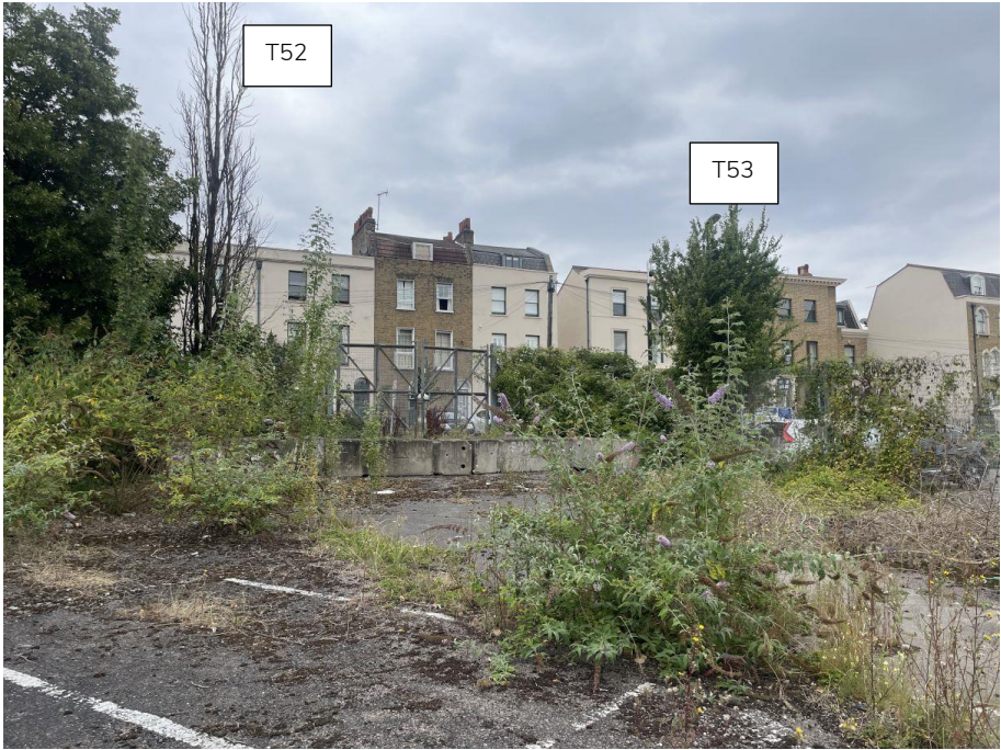
TC7. (14.08.24) looking west, T52 and T53 to be removed
