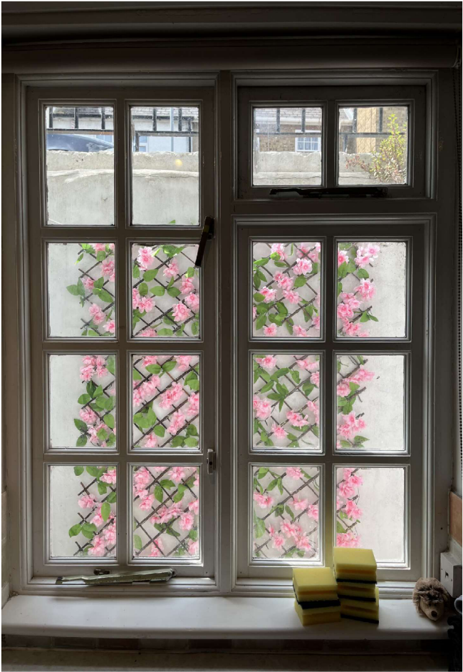
Existing Lightwell Window
