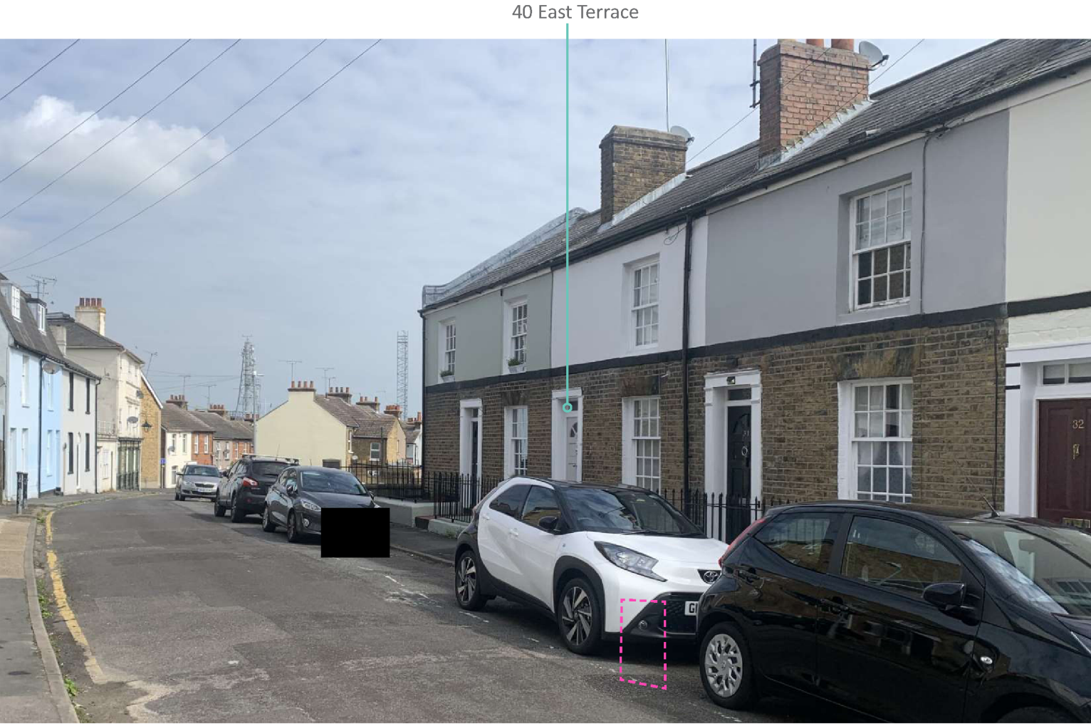
View of East Terrace looking north
