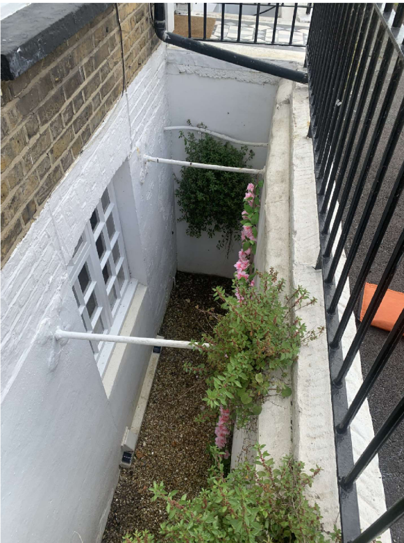
View of the existing lightwell
