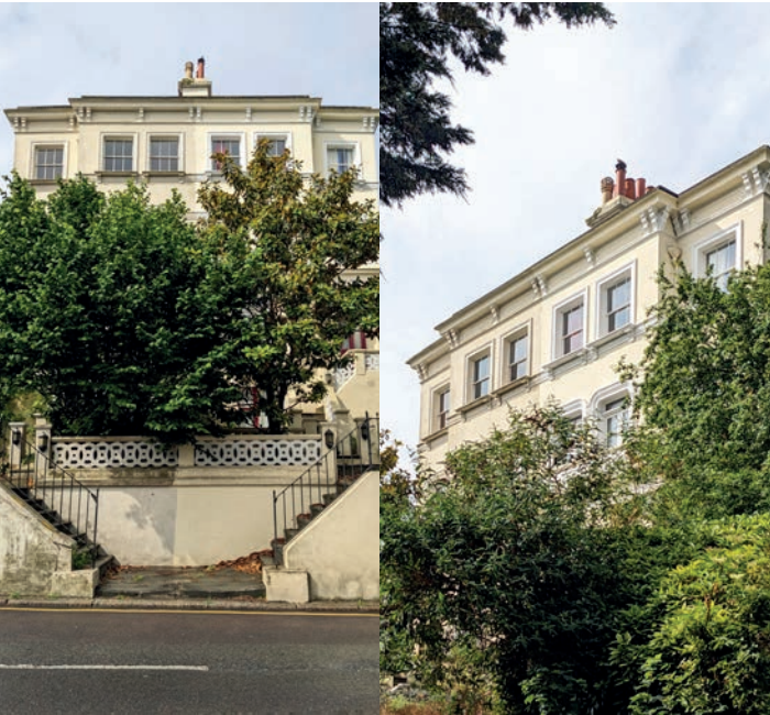
5-7 Parrock Road - Bronte Villas
