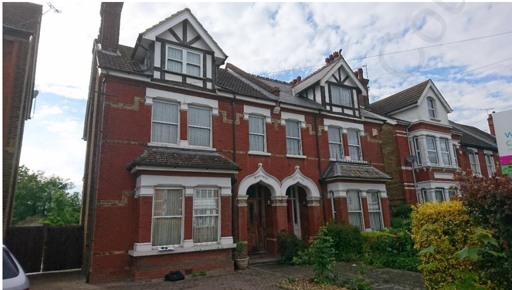
Front view of the property, showing no. 124 foremost with attached no. 122 and no. 120 further to the right.
