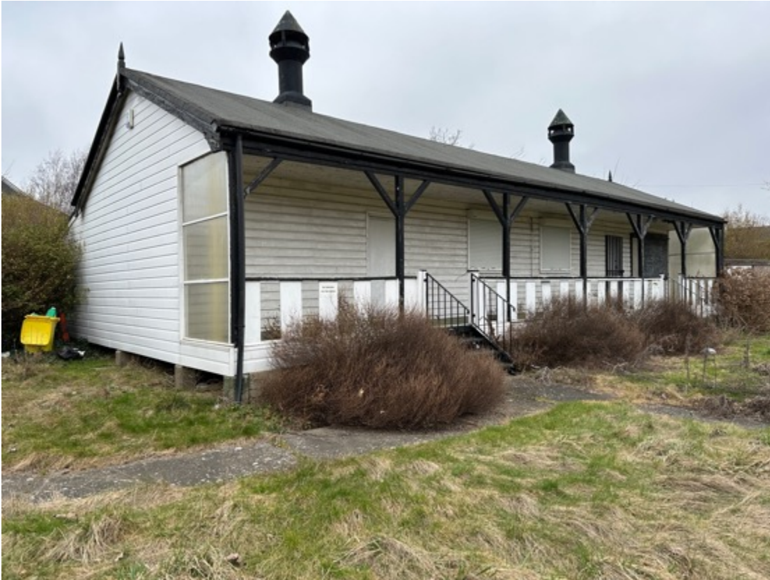
Photograph 1: Front of the clubhouse, looking north-west
