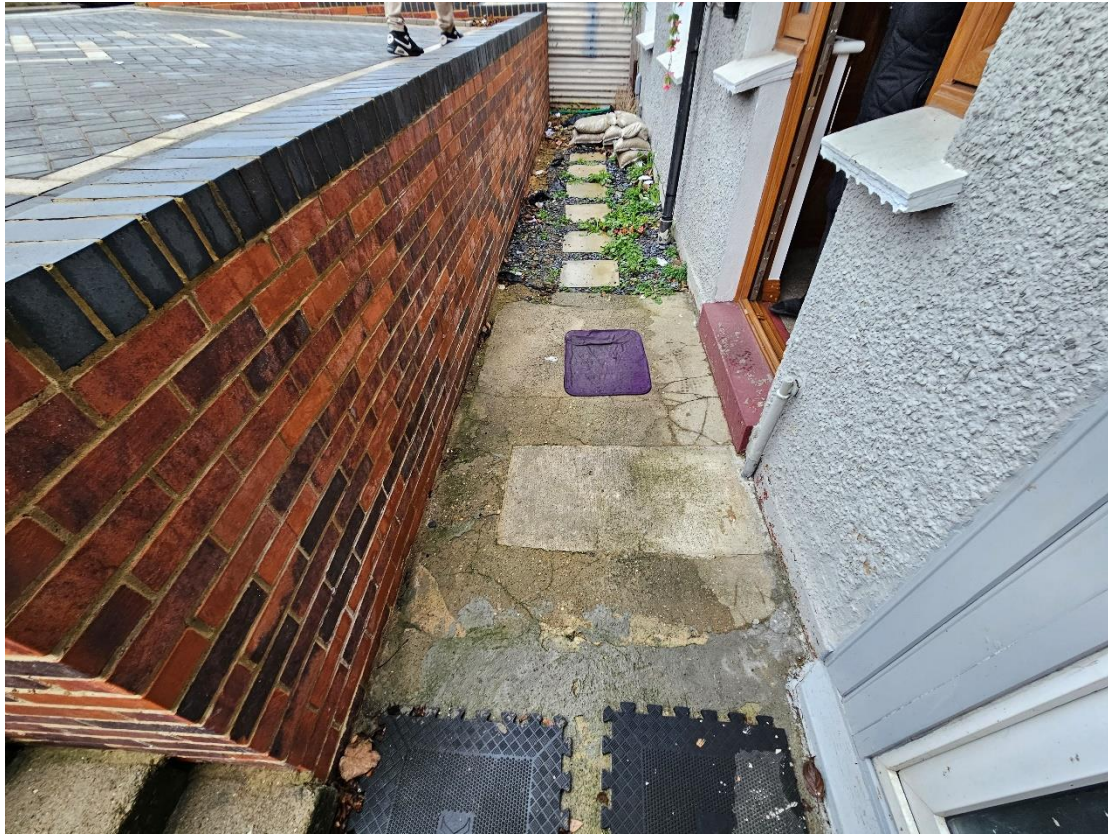
Fig.04 – Side access showing existing downpipe and permeable surface
