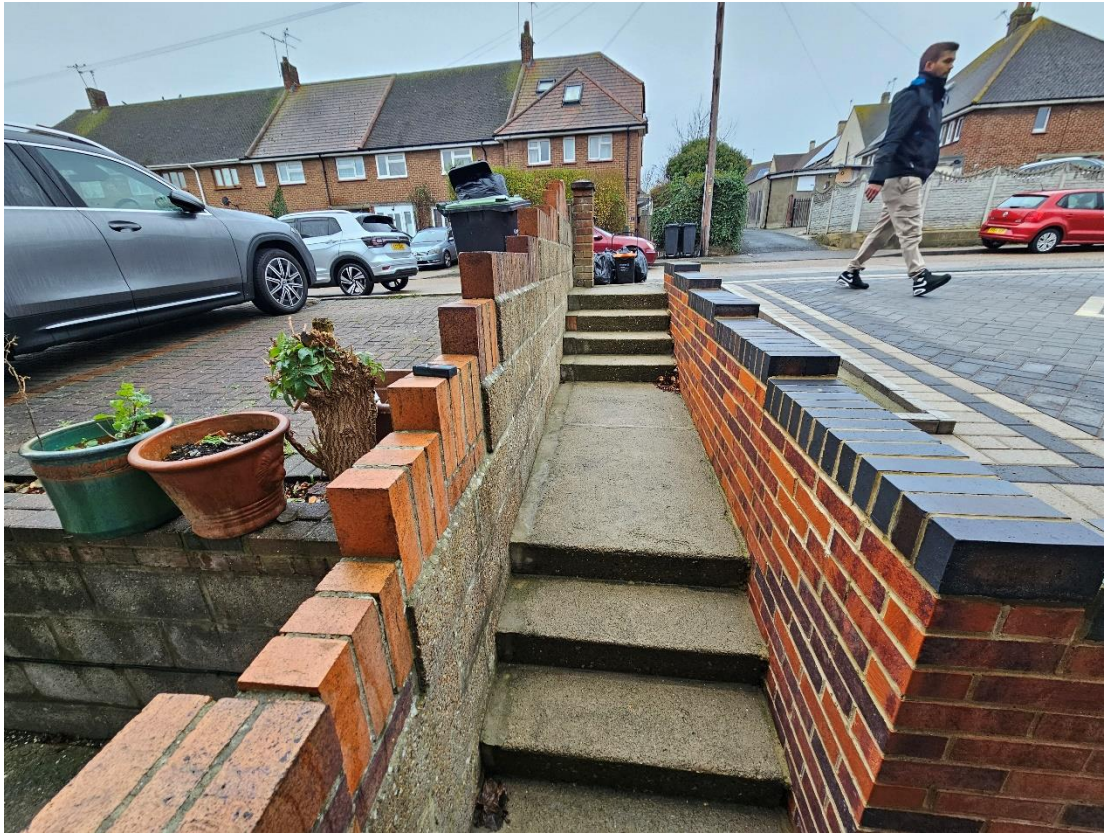
Fig.03 – Side access to property
