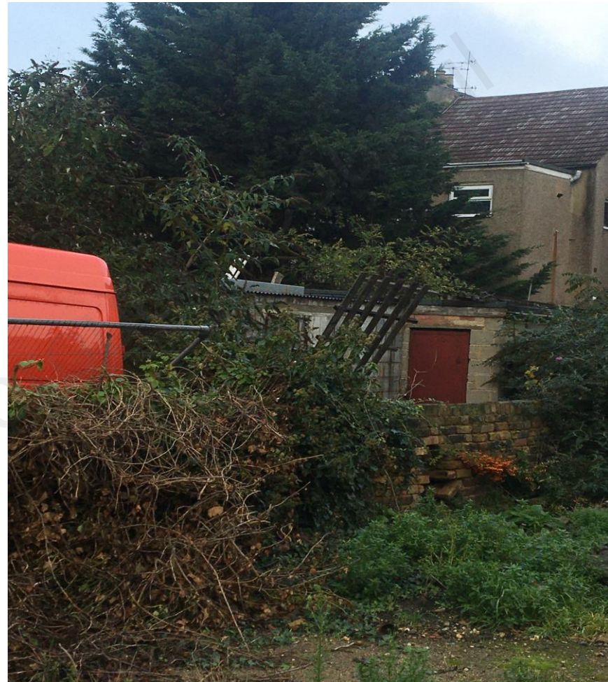
Photograph 4: Photo shows structure on-Site to be demolished.
