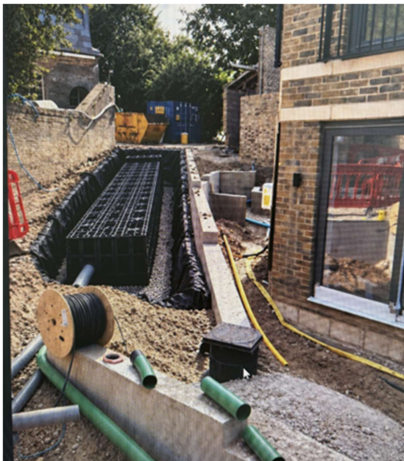
Figure 4-5 Installation of attenuation tank A
