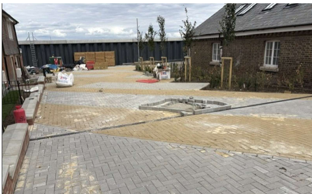
Figure 4-3 Channel drain traversing central access road.
