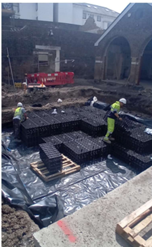
Figure 4-6 Installation of attenuation tank B
