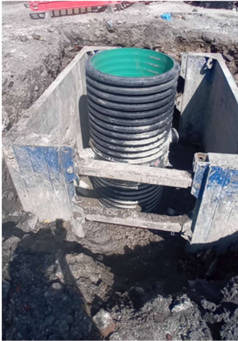
Figure 4-10 Installation of vortex separator.
