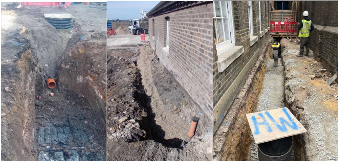
Figure 4-11 Surface water drainage runs during installation.
