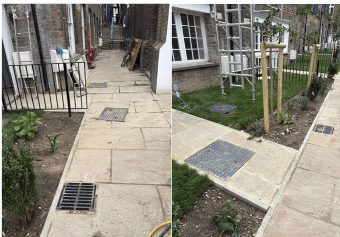
Figure 4-4 Manholes and gullies installed to units 12-19.
