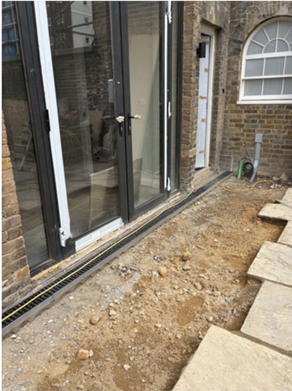
Figure 4.2 Channel drain during construction to side return of Unit 4.
