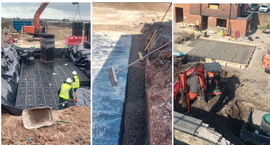
Figure 4-7 Installation of attenuation tank C, including backfilling and concrete cover slab
