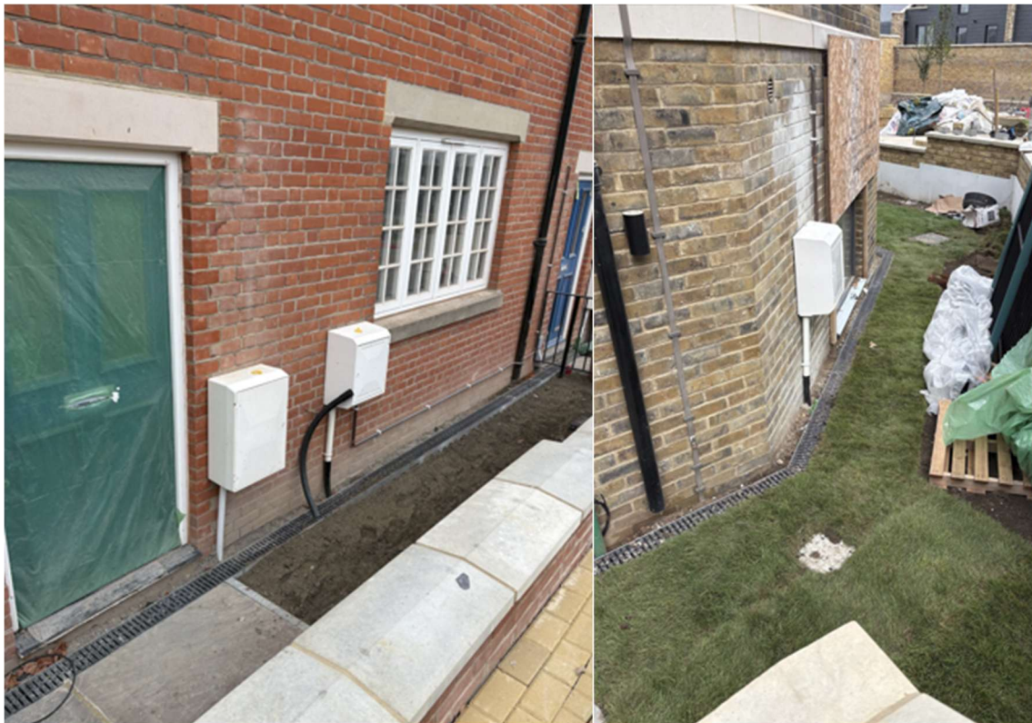
Figure 4-1 Channel drain and rainwater downpipe constructed along units 21 to 24 and to the rear of units 25 to 27.
