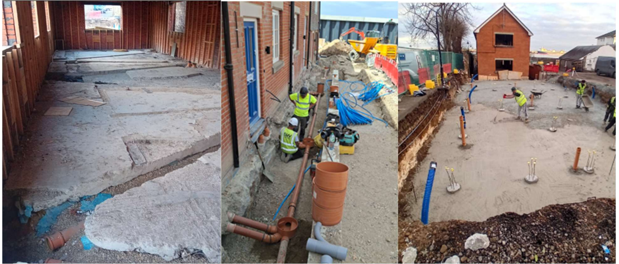
Figure 4-12 Foul drainage installation throughout site.
