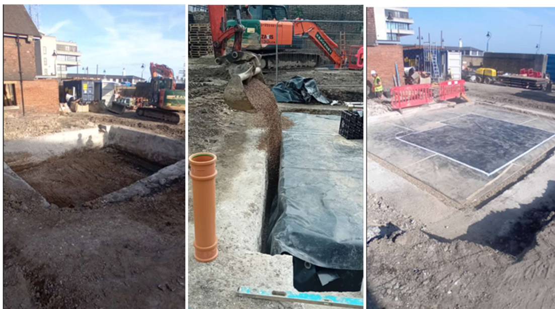
Figure 4-8 Installation of attenuation tank D, including base preparation, installation backfilling and completed membrane wrapping
