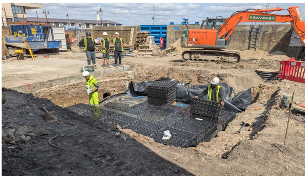
Figure 4-9 Installation of attenuation tank E
