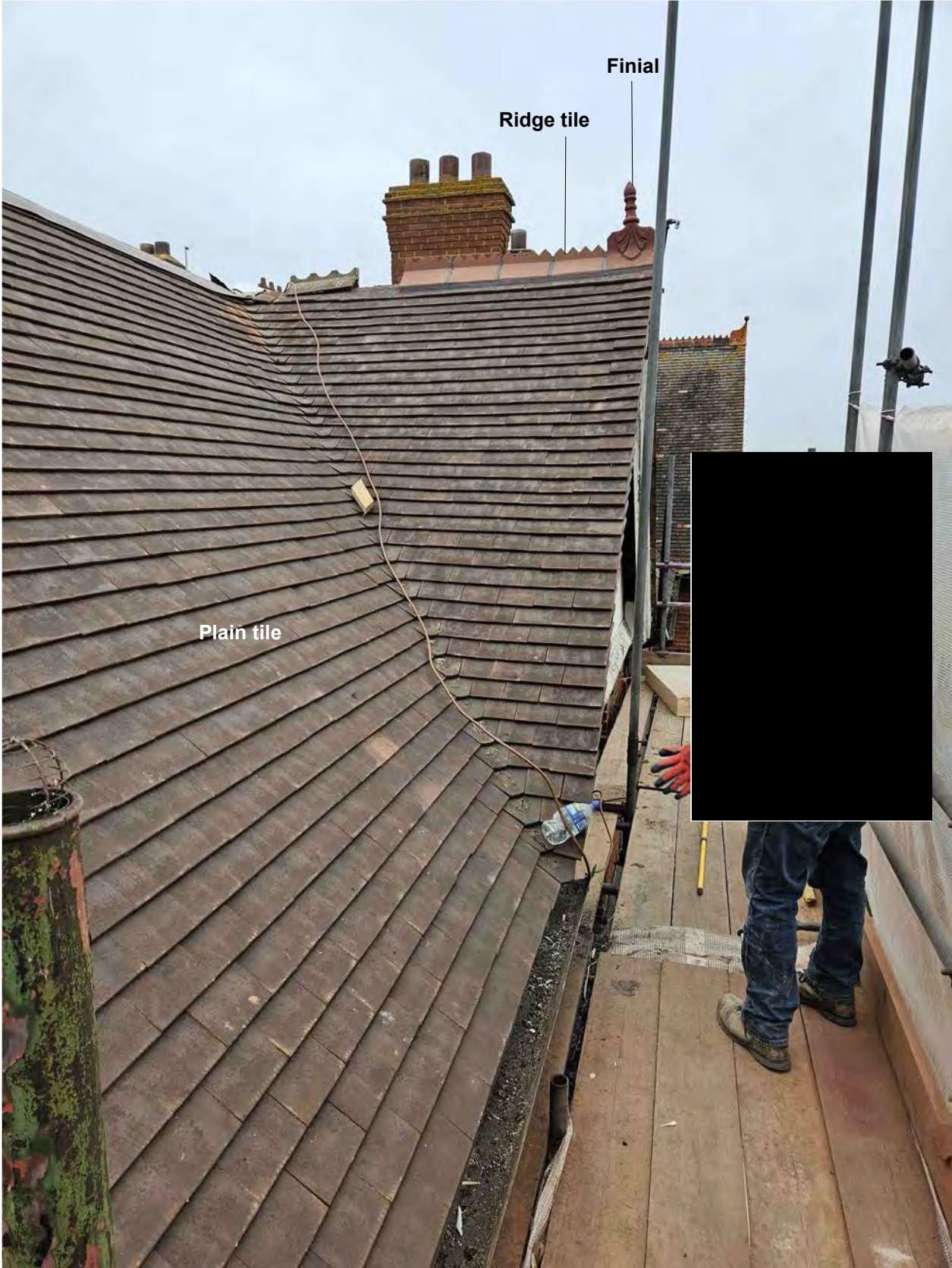
Finishes completed in 20240726
