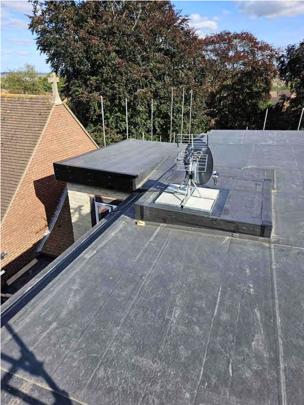
Finishes completed in 20240726
