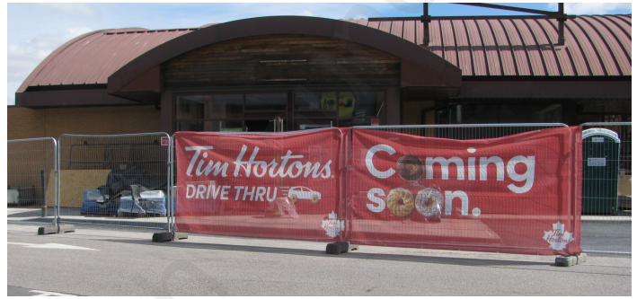
Photograph below under refurbishment August 2022
