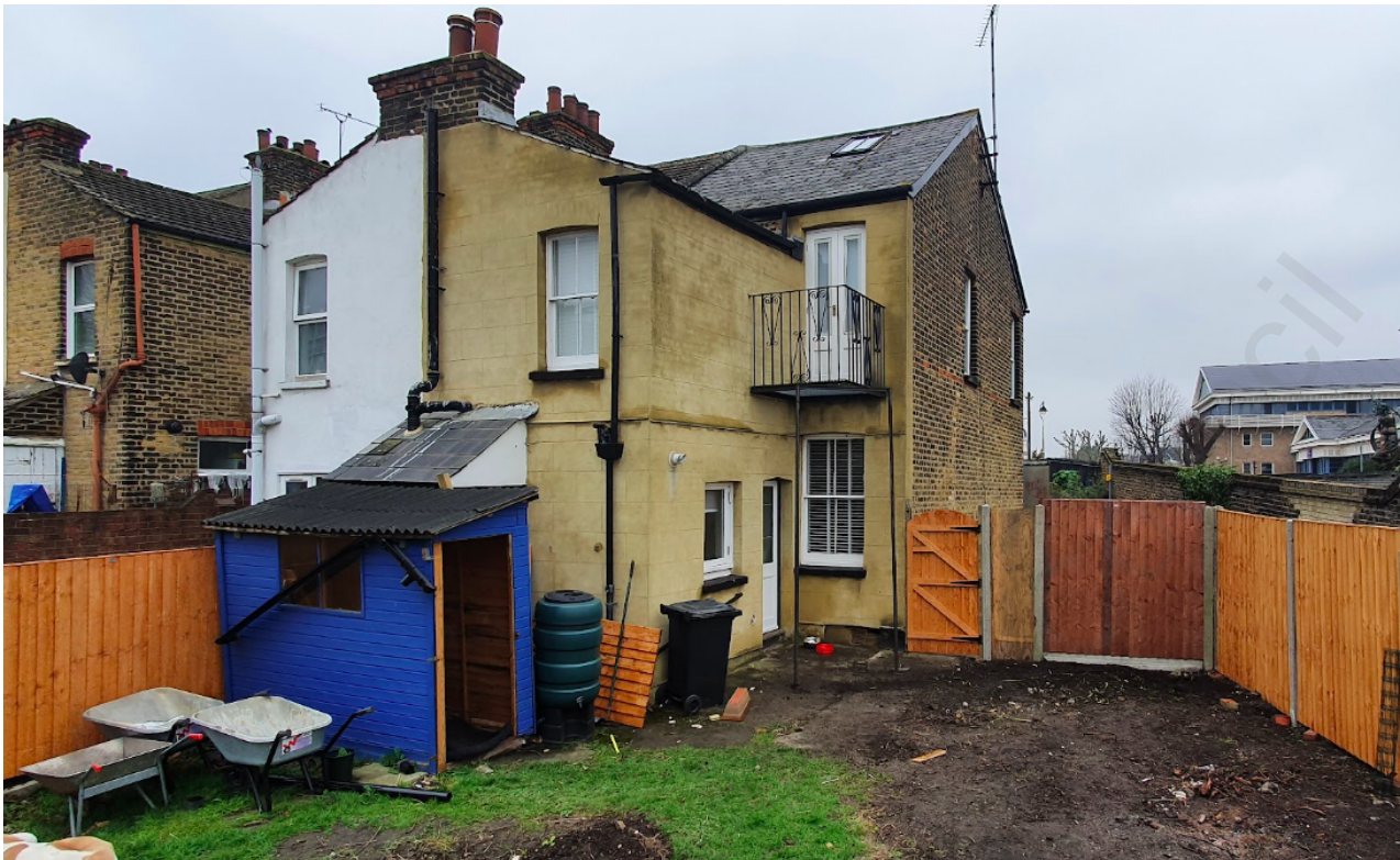
Rear Elevation of 18 Clarendon Rd, Gravesend, DA12 2BP, UK
