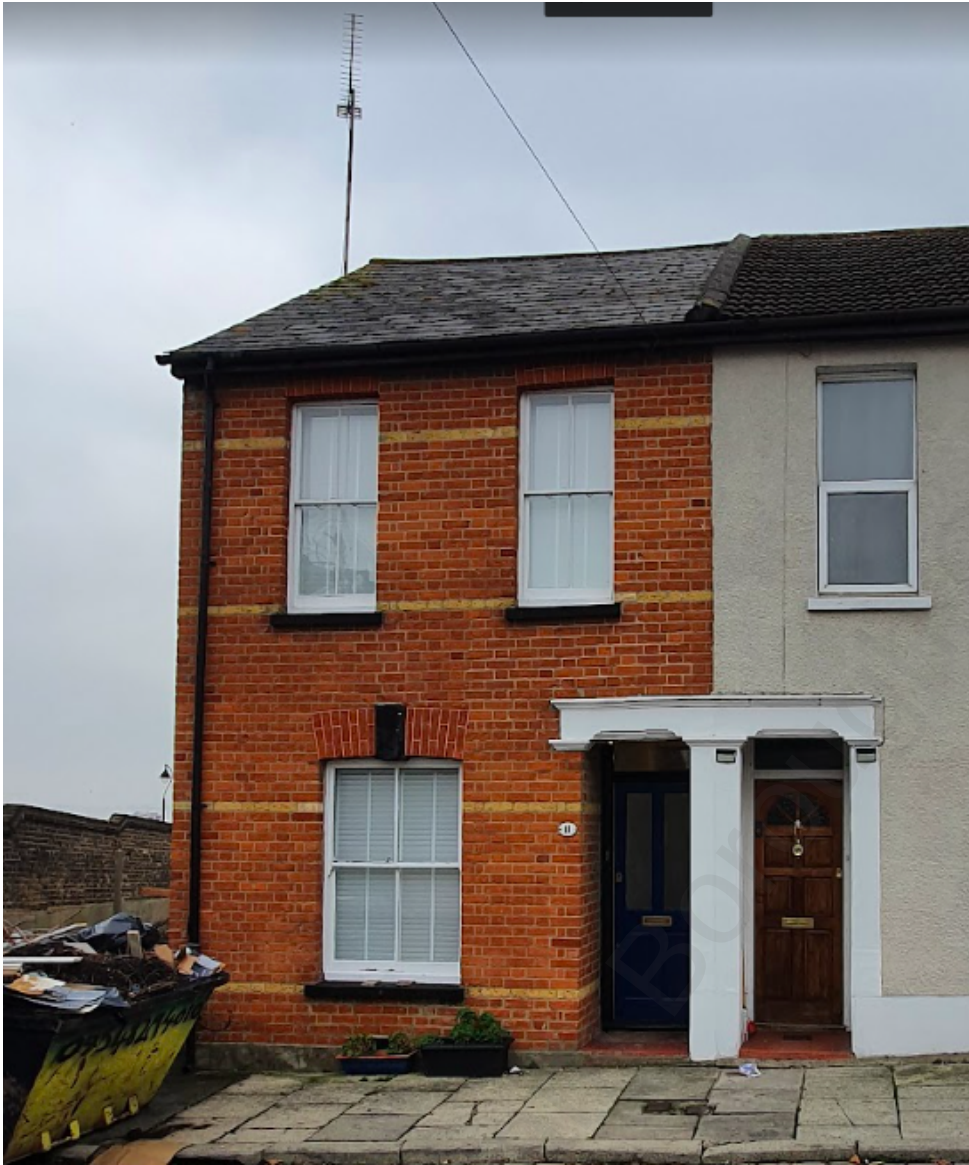
Front Elevation of 18 Clarendon Rd, Gravesend, DA12 2BP, UK
