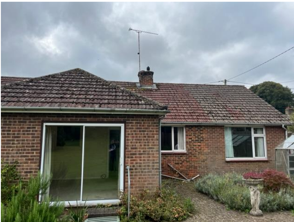
View of side and rear extensions
