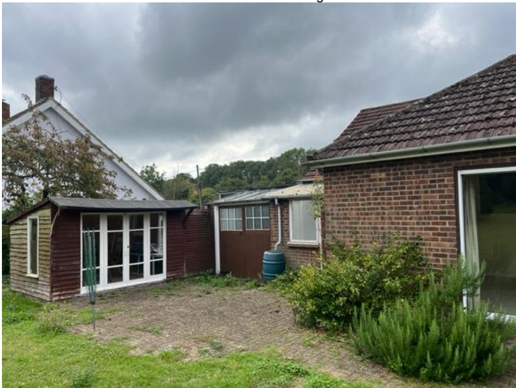
View looking towards rear of garage and summerhouse outbuilding (outbuilding to be retained)
