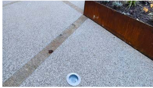
Figure 11. Resin Bound Surfacing
