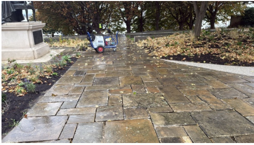
Figure 10. Yorkstone Pavers used in Phase 1.
