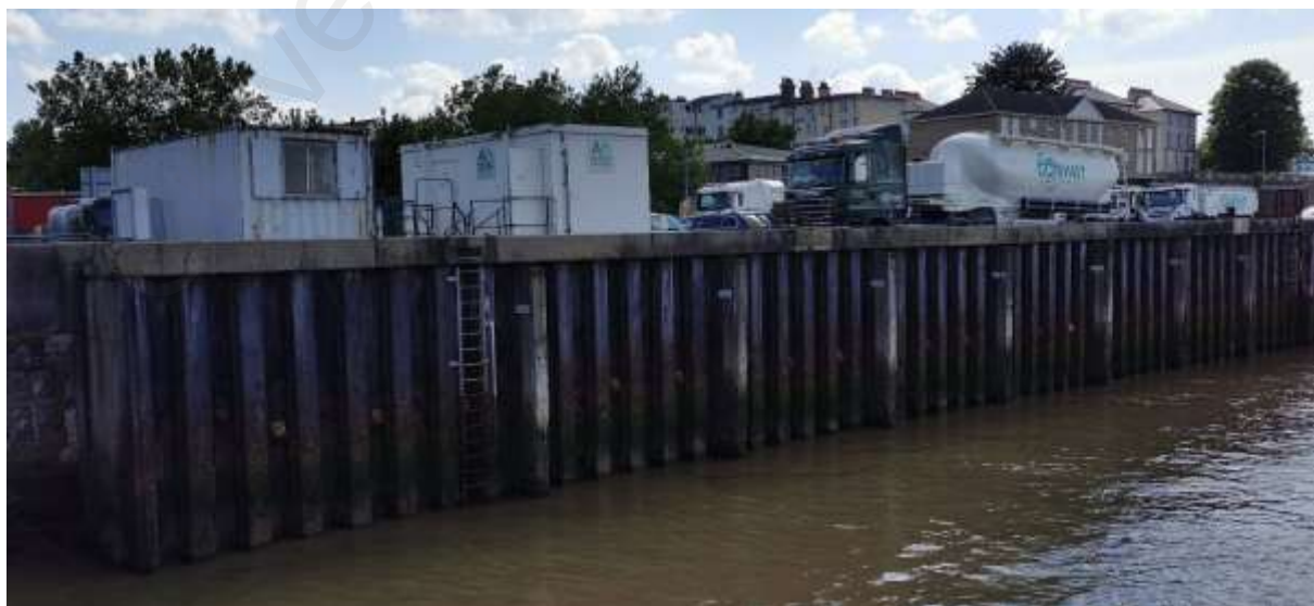
6. View showing piling river wall to west of wharfage
