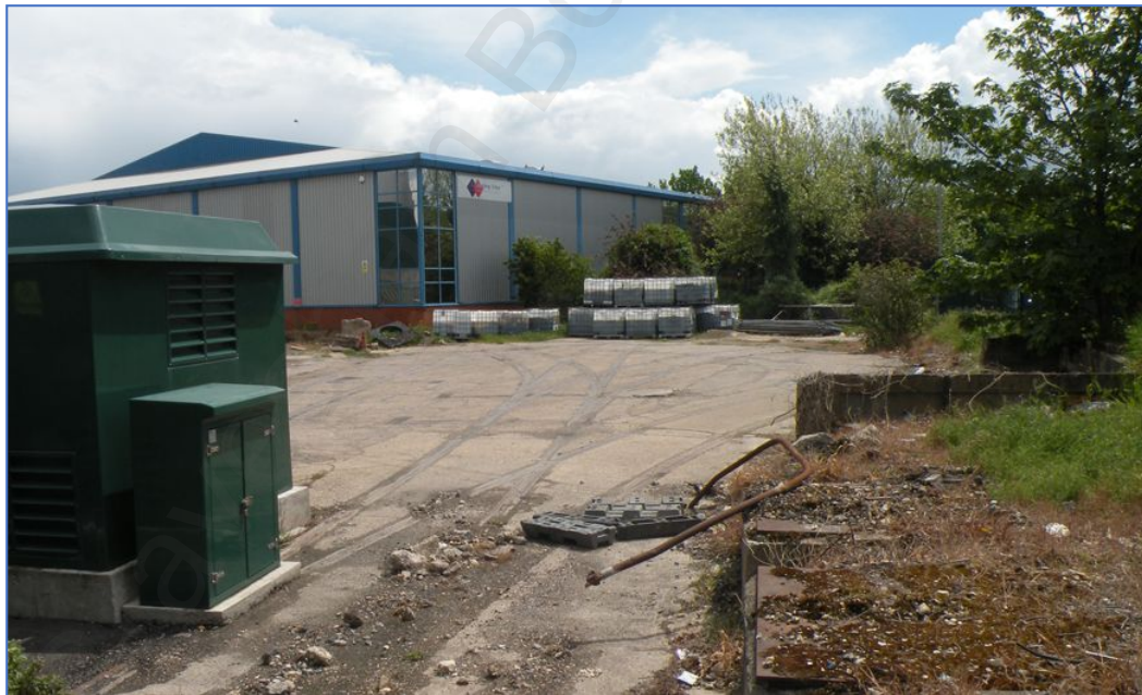
Figure 24 Looking south across PDA showing stub of walling (to right) and railway tracks
