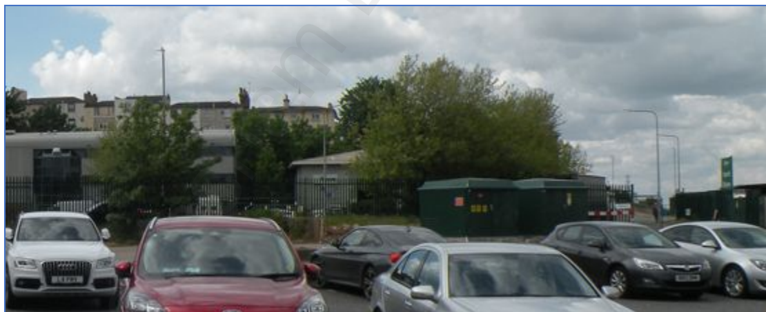
Figure 27 Looking towards listed quay walls from the PDA
