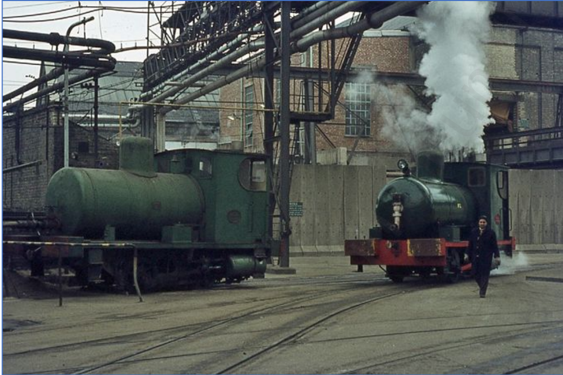
Figure 20 View south of the Imperial Mills, circa 1960s, approximate location of proposed bitumen tanks
