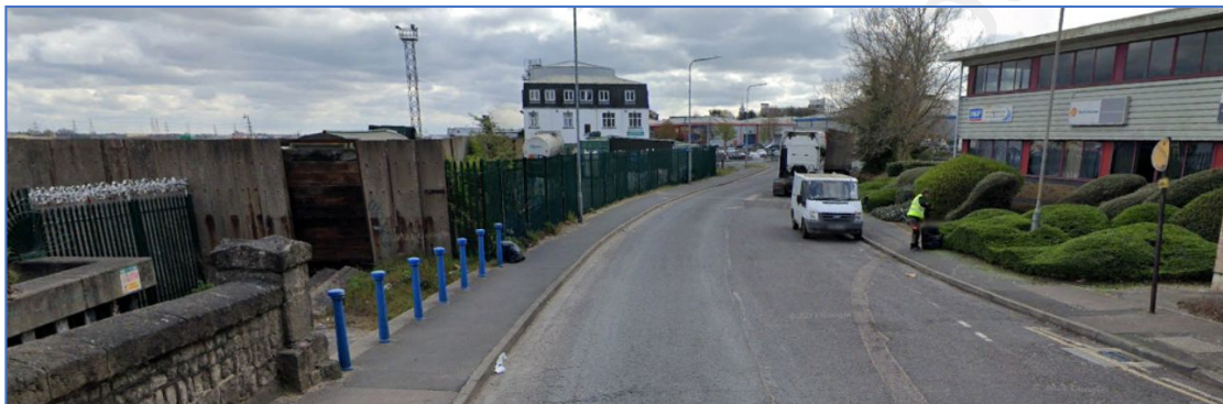
Figure 26 Looking towards PDA from eastern end of the listed quay walls
