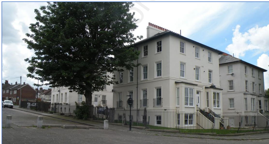
Figure 9 Recently refurbished buildings in Lansdowne Square
