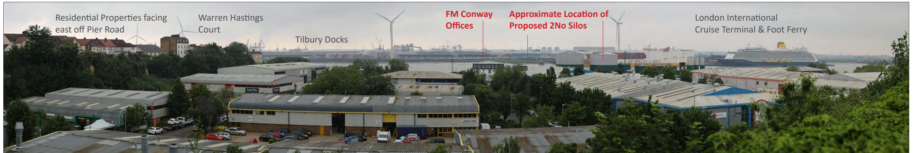
Receptor 16 - Receptor views from land around the W J King Vauxhall Gravesend car dealership, located off the A226 Overcliffe Road - staff and visitor have the opportunity to look north over the Business Park, down onto the Site at a distance of ~120m
