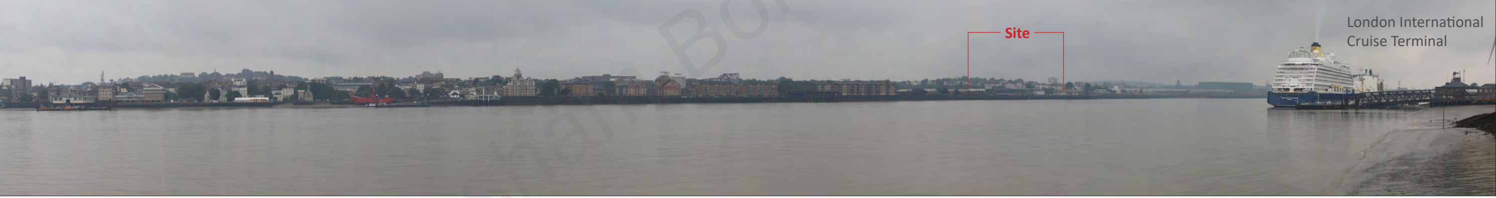
Receptor 3 - Receptors / visitors / setting of Tilbury Fort - looking south east towards the Site at a distance of ~1.3km
