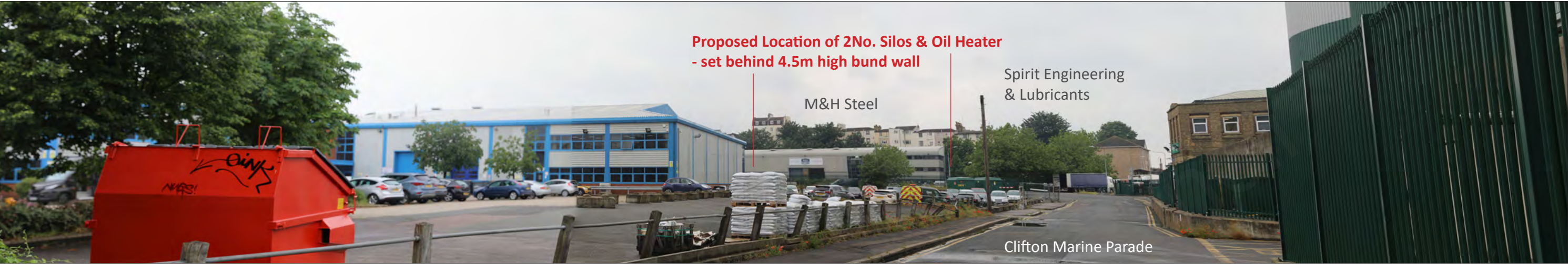
Receptor 10 & 11 - Users of Clifton Marine Parade - located within the Site AND Users of Site adjacent industrial units and associated car parking - looking north towards the Site at a distance of 0 to ~50m
