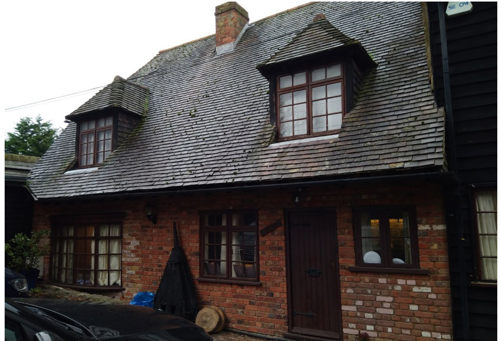
Fig.1 Old Forge - Front Elevation and Entrance
