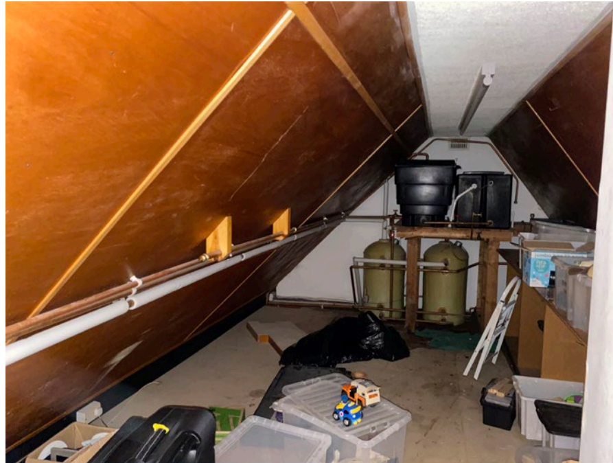
Fig. 15 - Photo of the loft space under the main clay tile roof.
