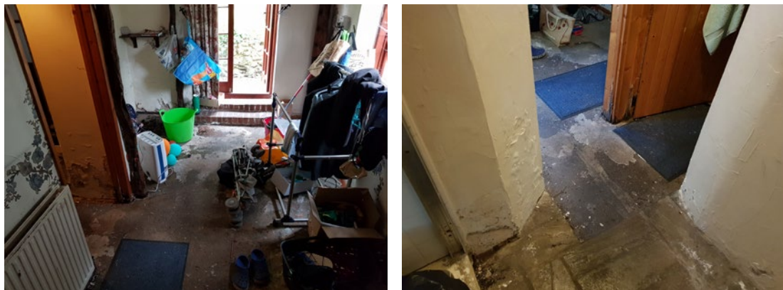
Fig. 16 - Photos of the existing ground floor.
