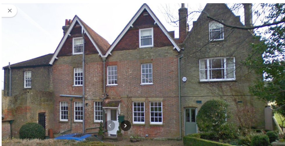
Front façade as seen in Google Street View images from 2009, highlighting the complete degradation of the façade over time.
