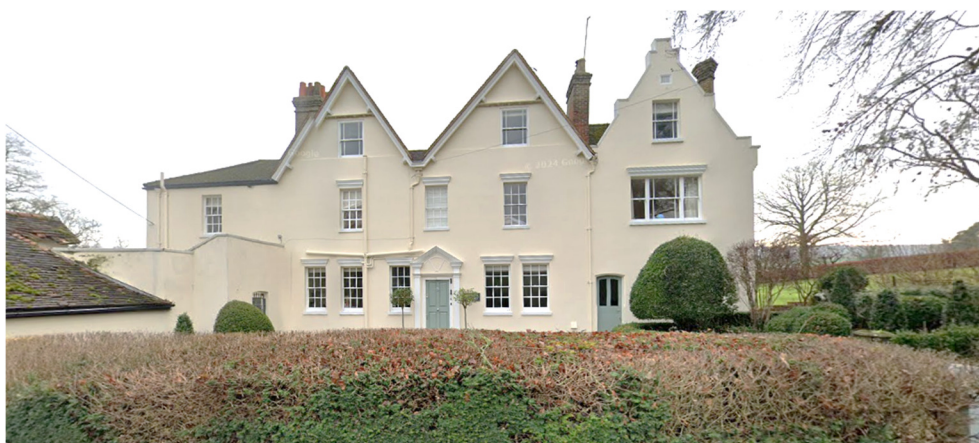
Window variations are also evident on the front façade, shown above in its current, rendered state.
