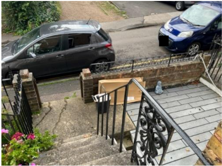
View from the house showing existing front wall, topped with railings.
