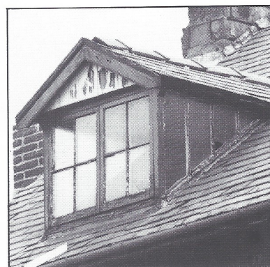
A dormer with pitched roof and glazed cheeks. Buxton, Derbyshire
