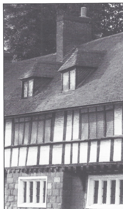
Dormers with hipped gables on a timber-framed building. Coventry, West Midlands
