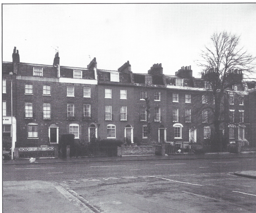
Early nineteenth-century terrace houses with a single flat-topped dormer centrally placed between the windows on the main facade. London Borough of Lambeth
