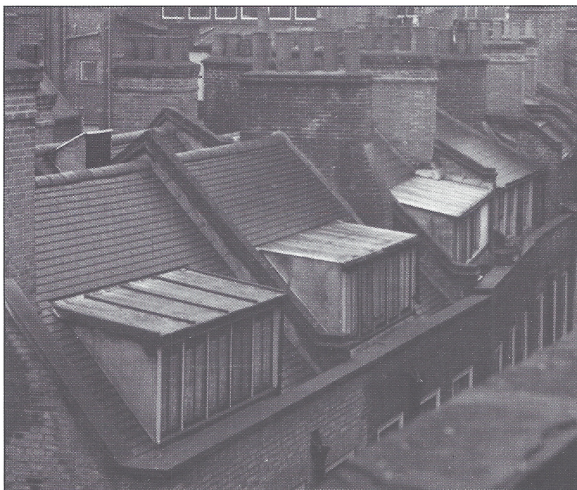
Five light dormers on houses built in the 1720s. These dormers are probably later alterations and were possibly added to provide well-lit workshop areas. They are not suitable additions to houses. Meard Street, Westminster
