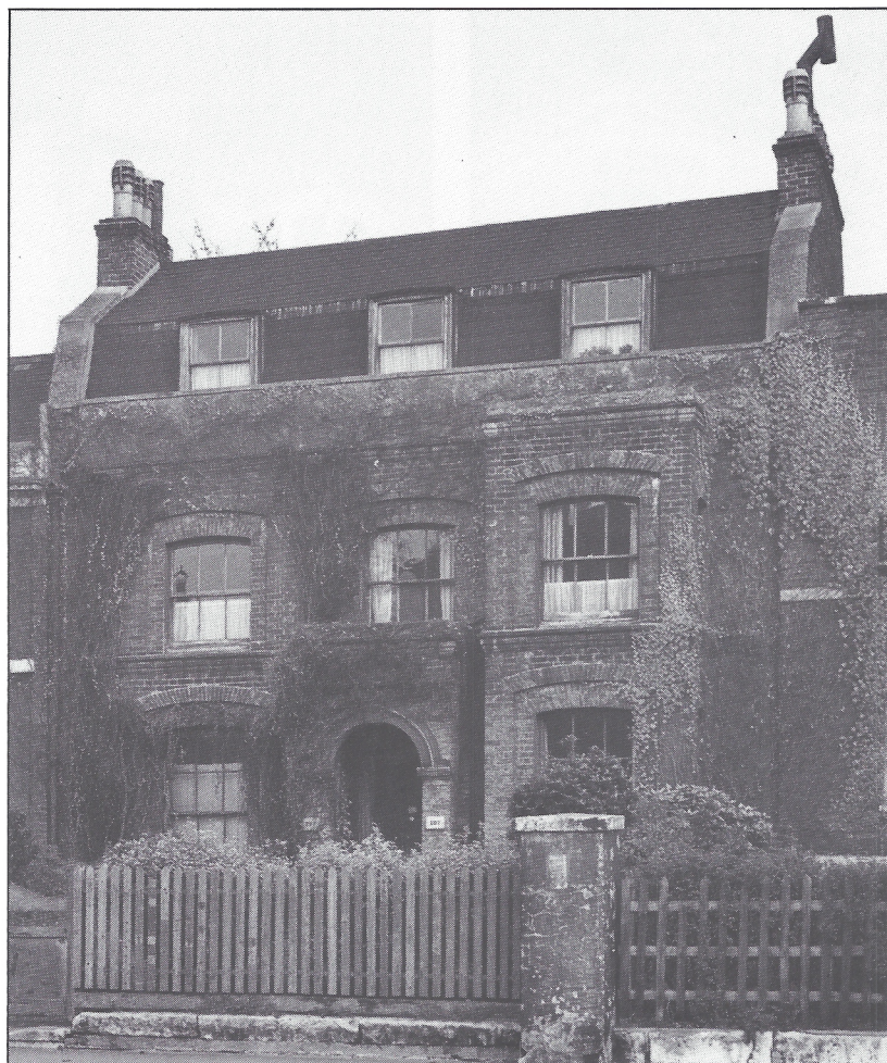
Dormers with double-hung sash windows in a house built in 1824. London Borough of Lambeth
