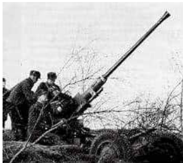
The 40mm Bofors Gun anti-aircraft gun could propel High Explosive and Incendiary shells up to 41,000 feet.
