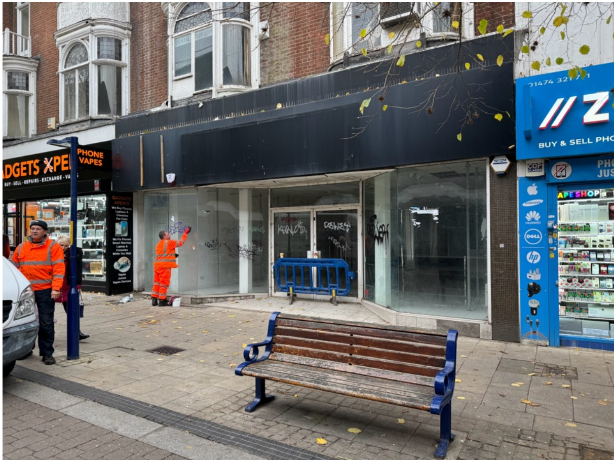
The application site
