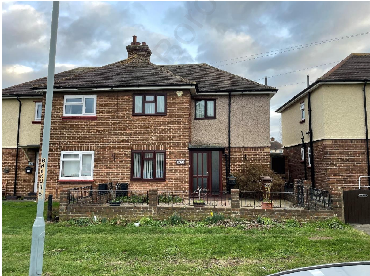
Fig 2.1 Front of No 55 Harden Road
