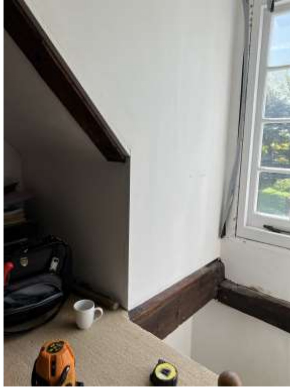
Image of existing dormer window, internally.
