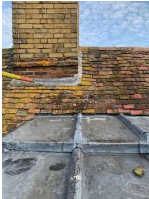
Image of chimney stack above roofline and existing dormer roof.
