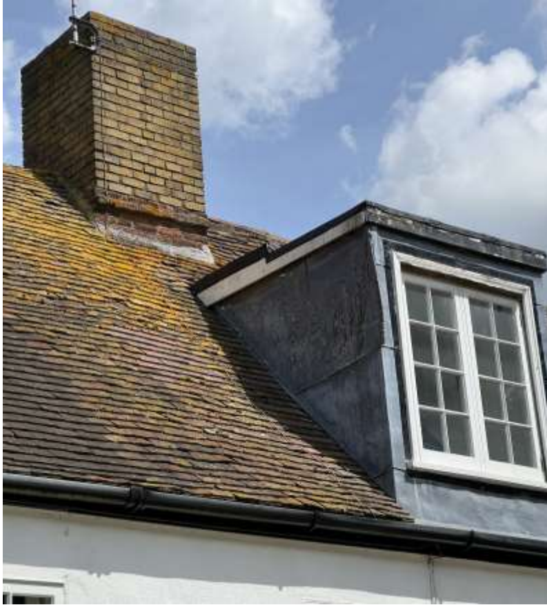
Image of chimney stack above roofline and existing dormer window.
