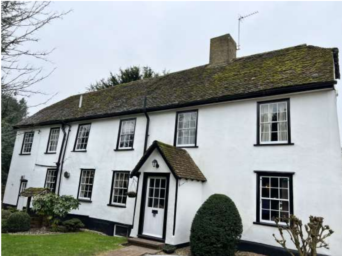
Image of the front (north) elevation.
