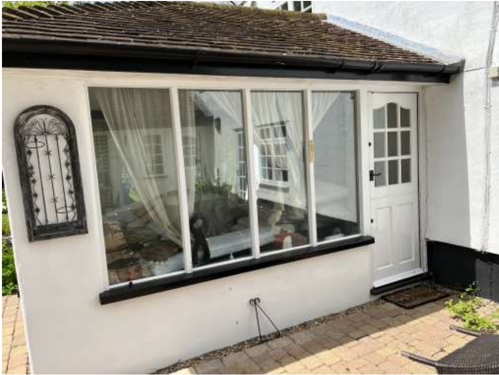
Image of the east-facing elevation of the modern extension at the west end of the rear elevation.
