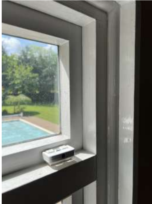
Internal image of the storm-proof windows to the rear elevation.
