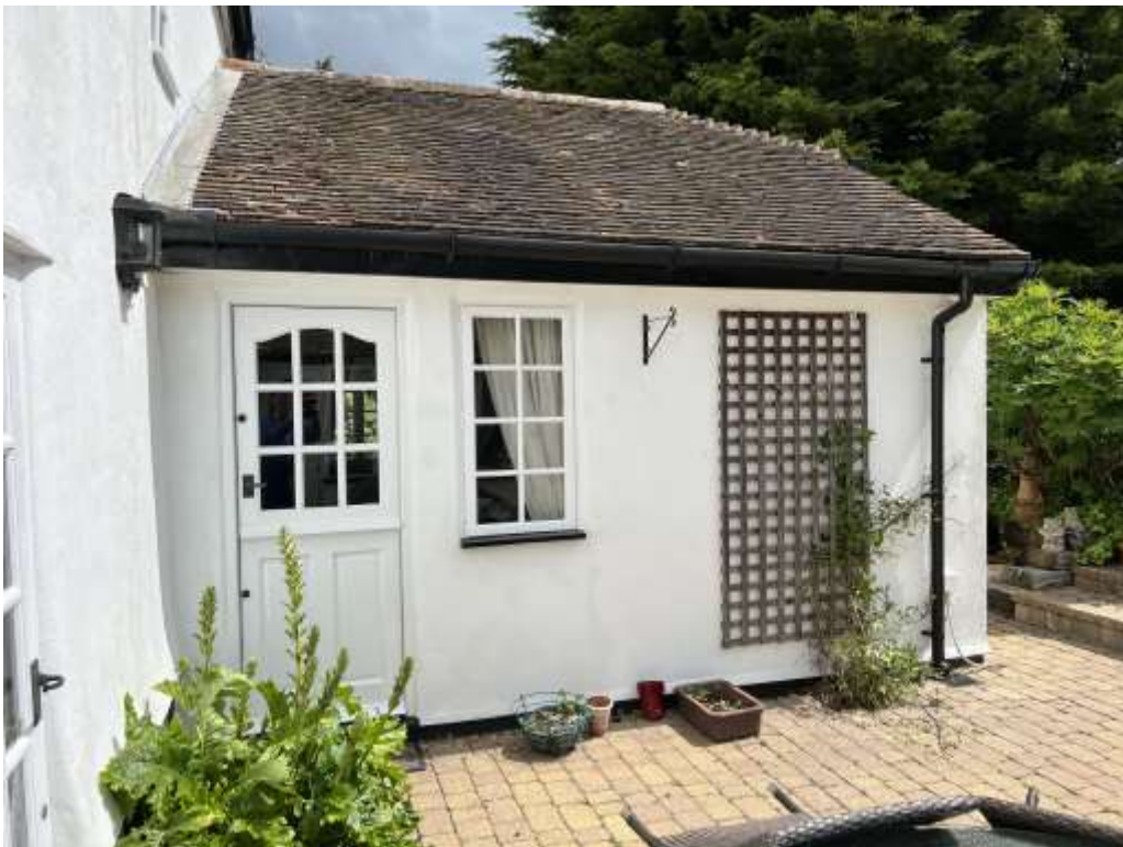
Image of the west-facing elevation of the modern extension at the east end of the rear elevation.
