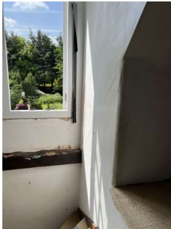
Image of existing dormer window, internally.
