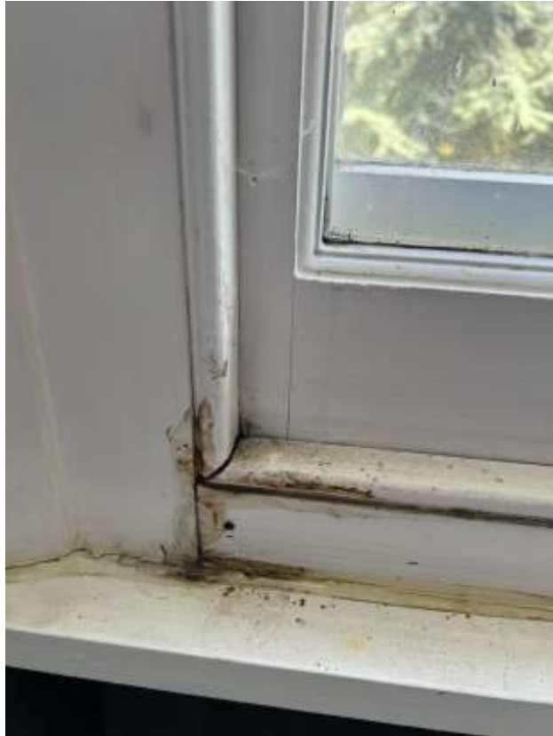
Internal image of the sliding sashes to the front elevation.
