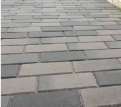
Permeable vehicular sett paving,
