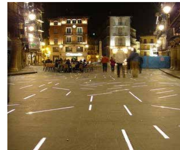
Lighting incorporated into paving
