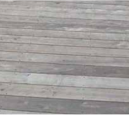
Composite timber decking
