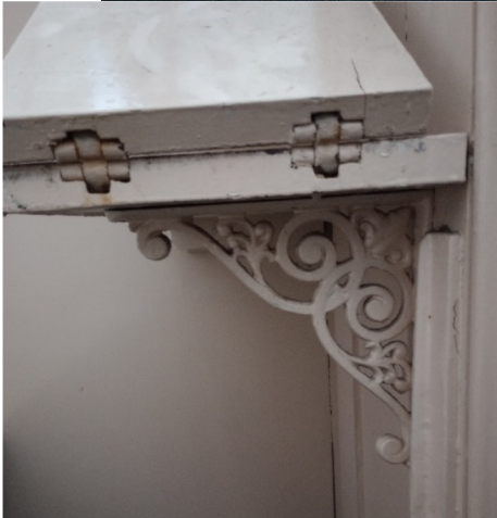
Boxed enclosures against West wall & hinged shelf and cast iron support bracket to box accessed from podium.
