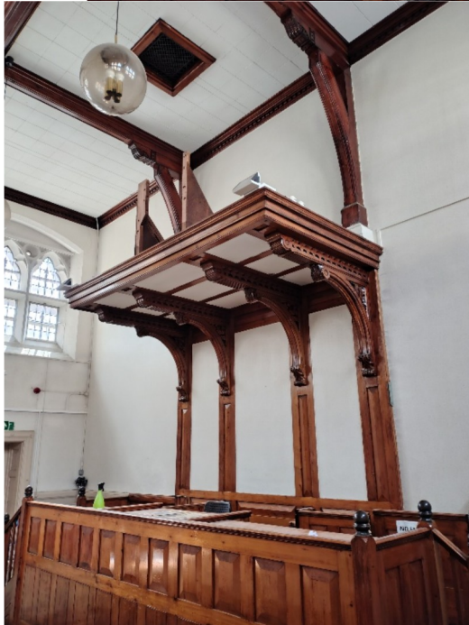
Close-up views of panelling to Judge's bench and soffite of canopy over the bench. The vertical brackets, above the canopy, were to support the royal crest now removed
