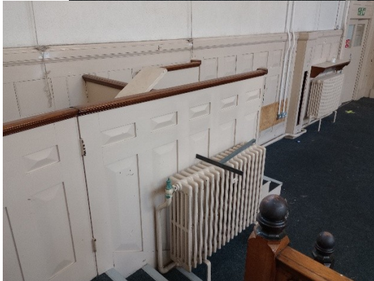
Box abutting West wall of Court Room.
