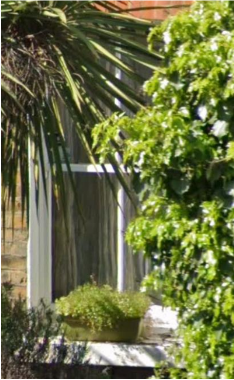
Close up of ground and first floor level
