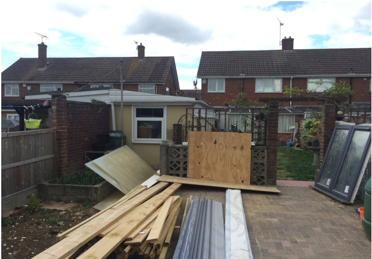
At rear of back garden looking towards the east at the front
