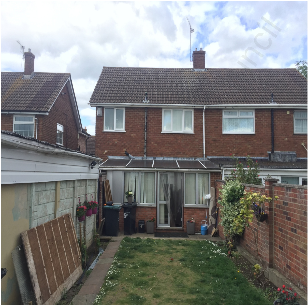
Rear West Elevation as seen from the back garden
