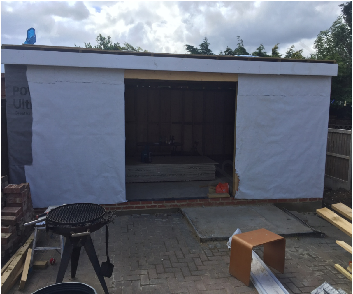
Front East Elevation of New Out Building
