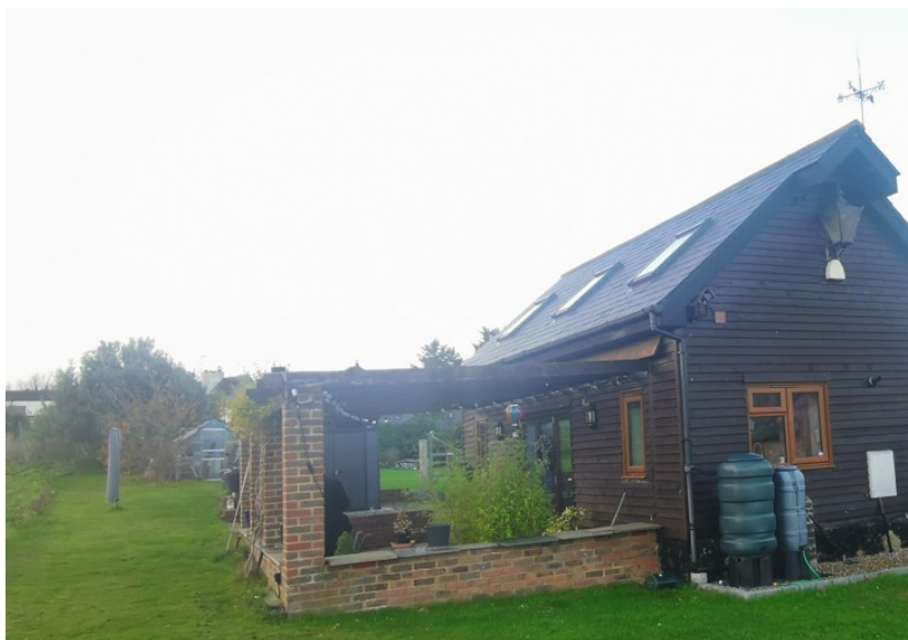
P002 – Existing attached pergola
