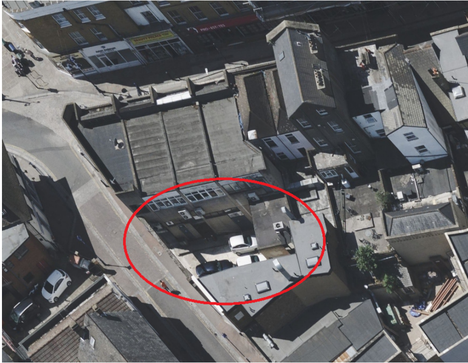
Fig 02 – aerial view rear service area 21 – 21c King street
