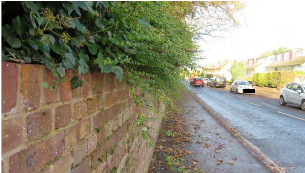
Photo 2: Looking north-west along Downs Road near the proposed access
