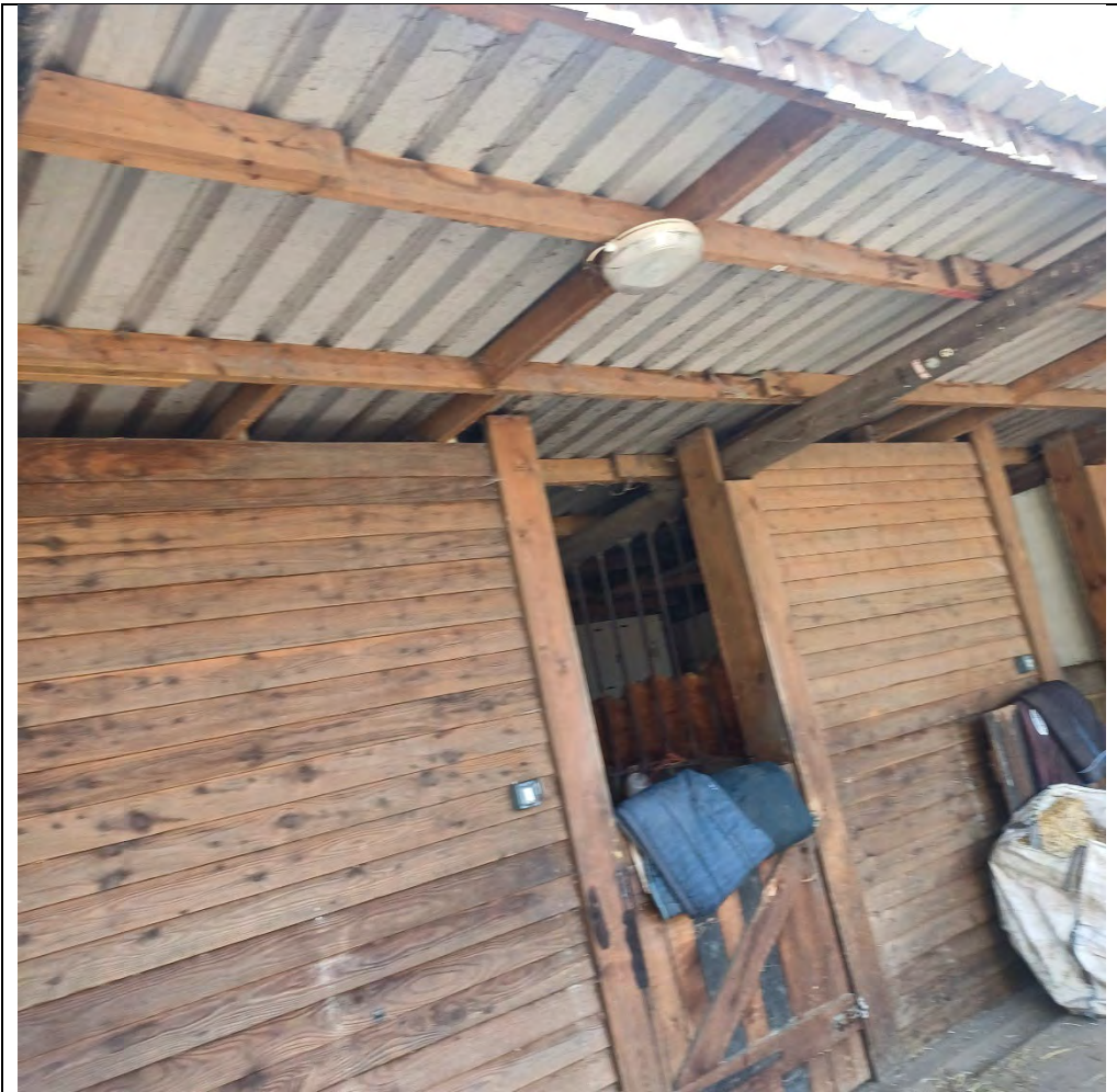
Plate 6: Suspected asbestos cementitious sheeting on main site
