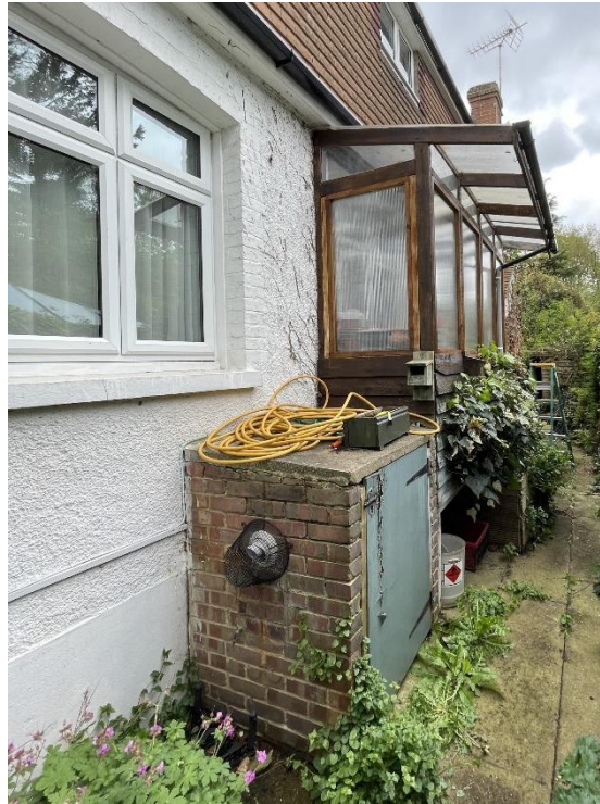
Fig 009 – To be demolished: lean-to structures at the side of no.29 Manor Road
