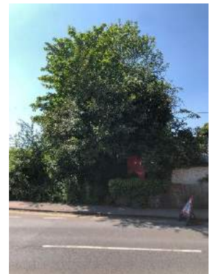
Overgrown planting at The George Inn to be trimmed/removed to enhance vista to the Listed Building
