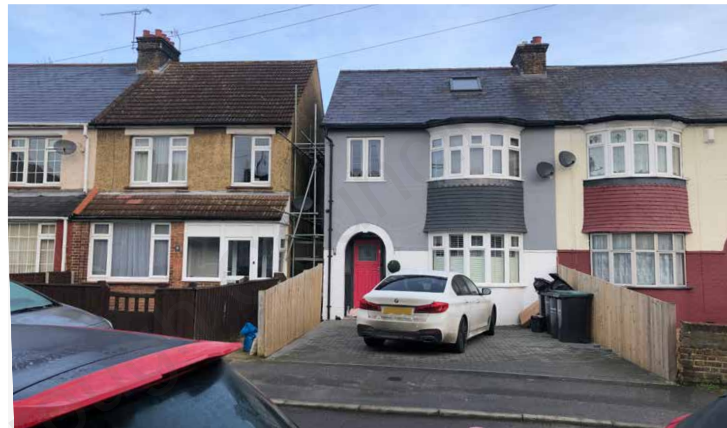
View 09 - A house on Waterton Avenue that has had similar alterations, including a dormer to the rear, Hip to Gable roof alterations.
