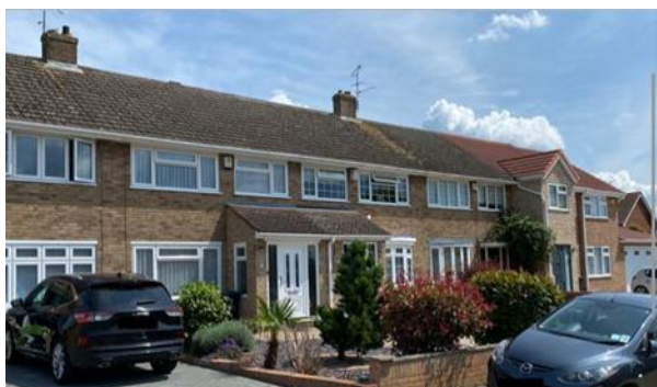
Terrace containing the application site
