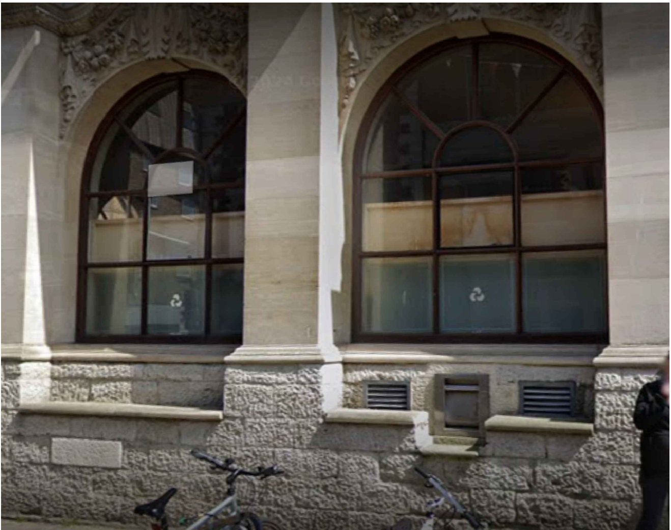
01 EXISTING ELEVATION PHOTO NTS
