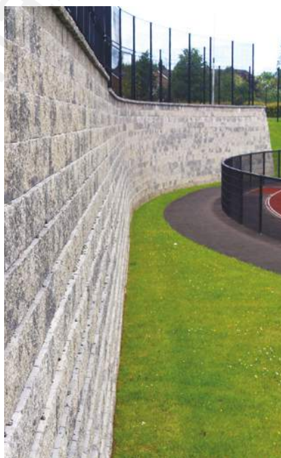
Walling & Retaining Walls
