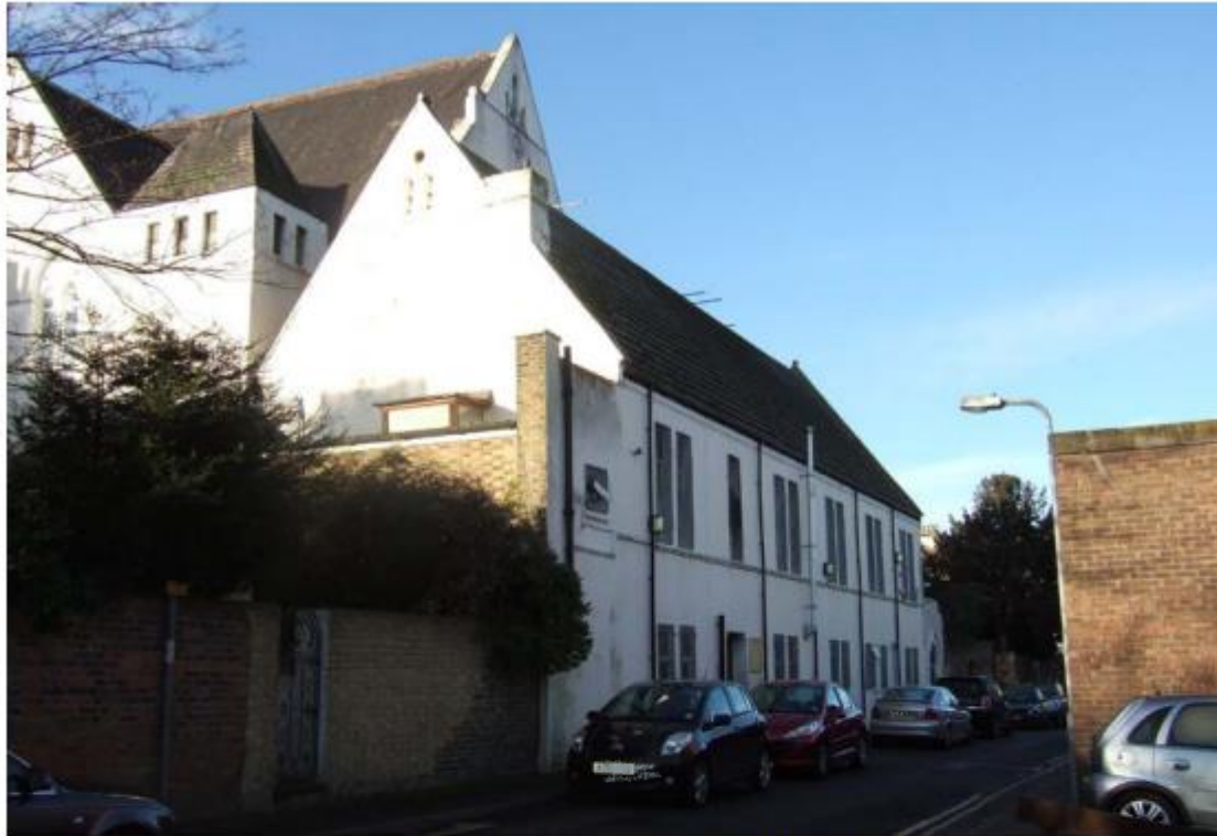
□ REAR SECTION OF EXISTING BUILDING FRONTING WILLIAM STREET
