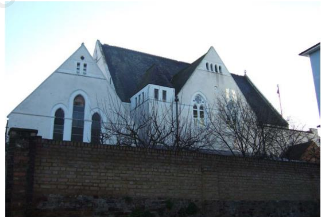
□ WESTERN FLANK OF EXISTING CHURCH BUILDING
