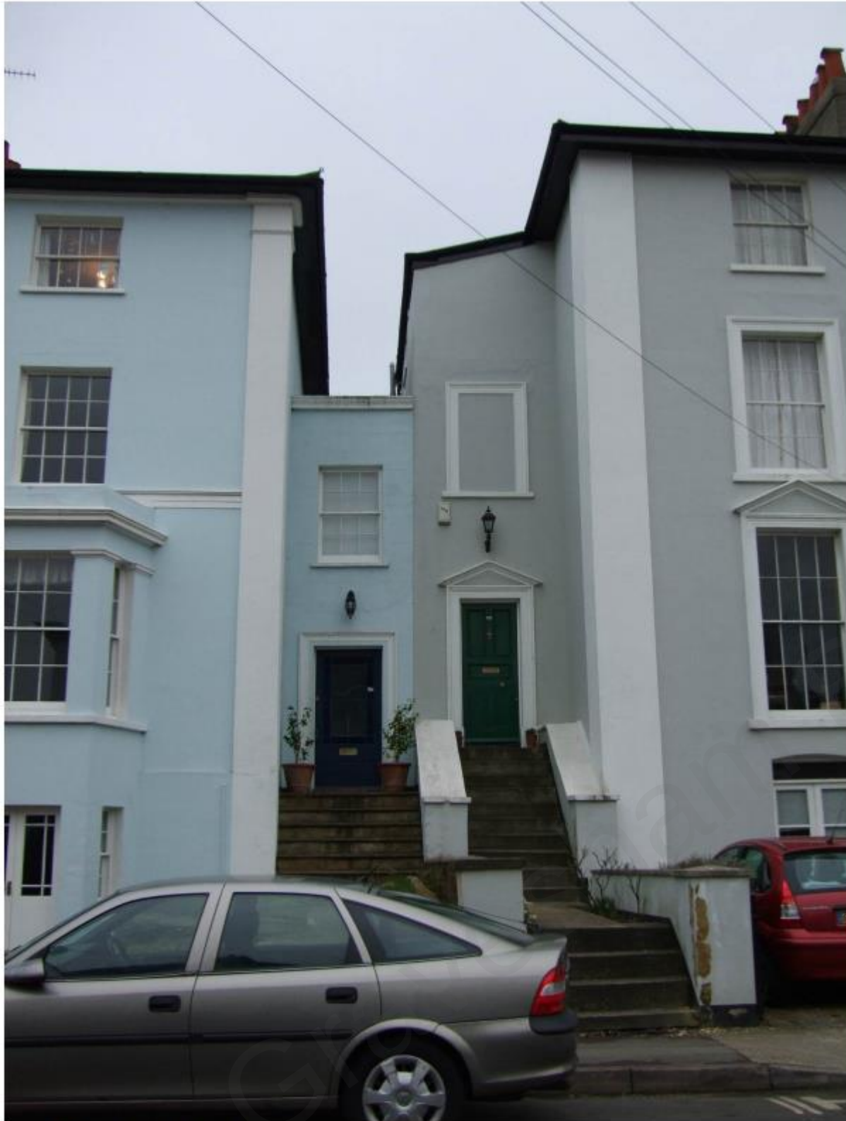
□ ENTRANCE TO 32-35 CLARENCE PLACE
