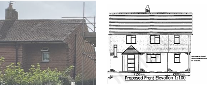
number 6 roof extension adjacent continues the original roofline
