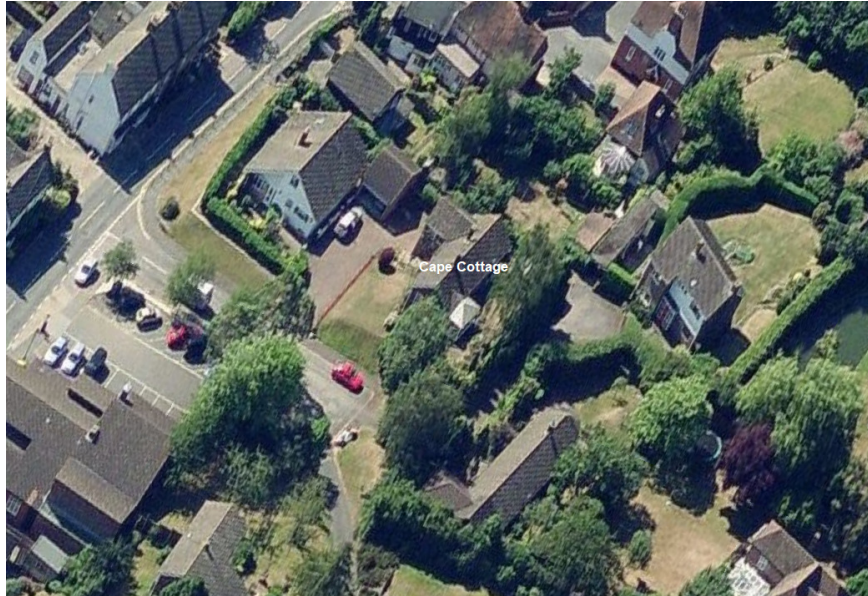
P001 – aerial view of site looking south
