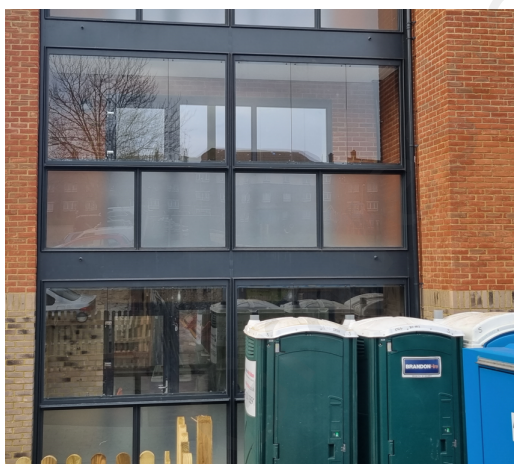
Ground and First Floor (Rear Elevation)
