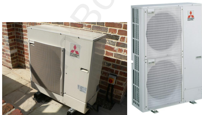
Figure 5: Mitsubishi example ASHP external fan units
